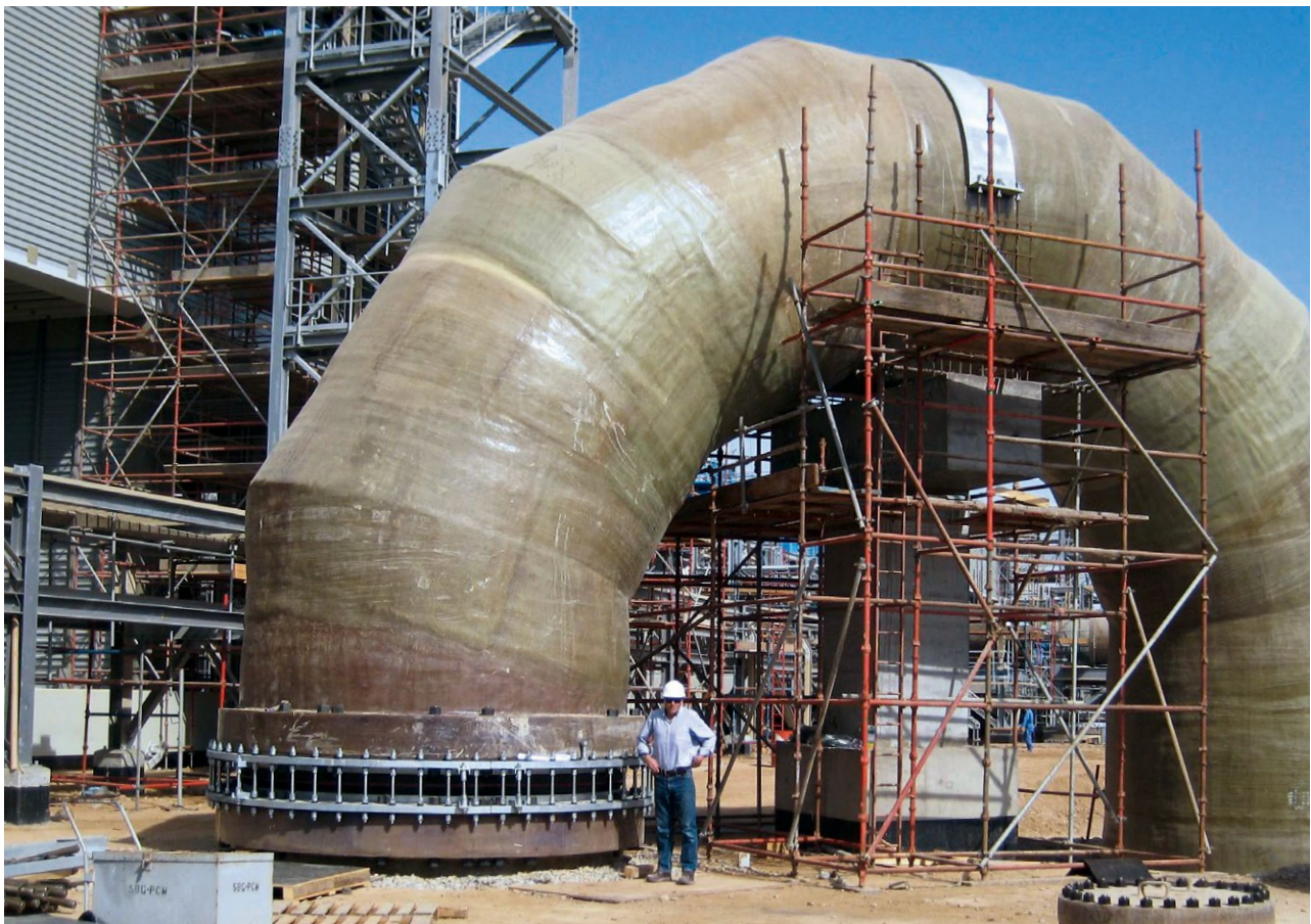
Large bore lateral rubber expansion joint, type U110M GRP pipe \varnothing 3,600 mm of a utility plant work-shop hydraulic test at 13 bar
