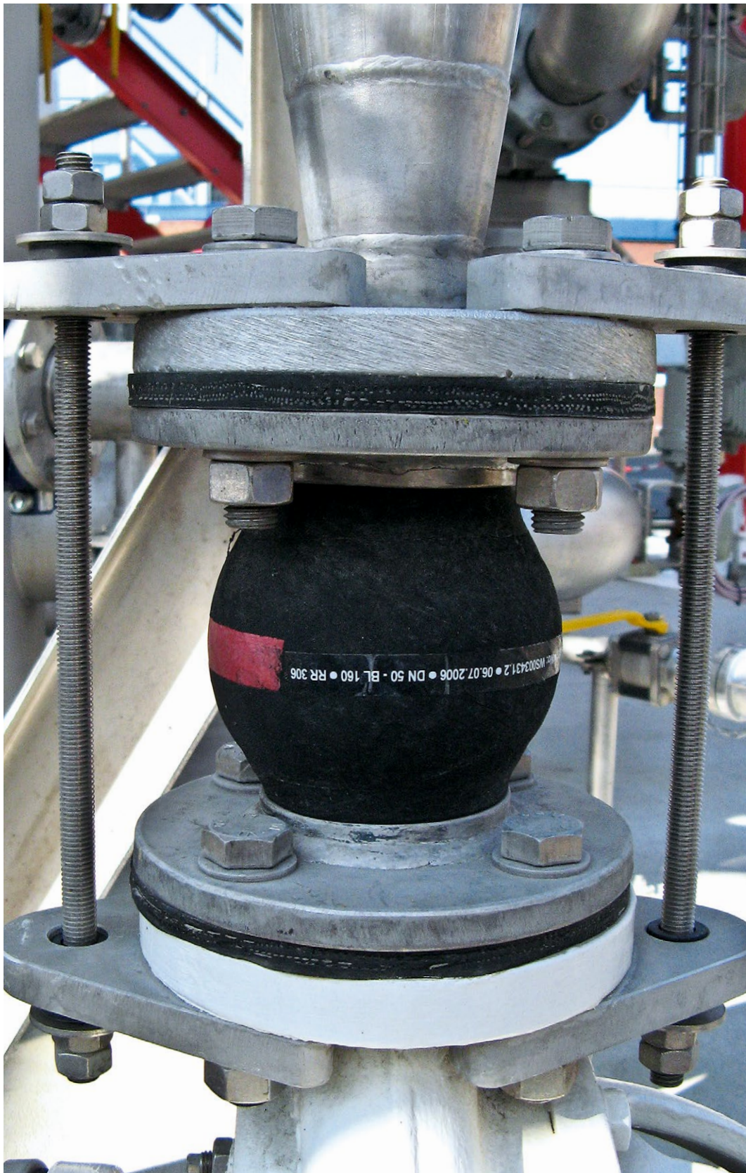
Lateral expansion joint, type U110R on the pump pressure side in a paper mill Ø 50 mm, 10 bar
