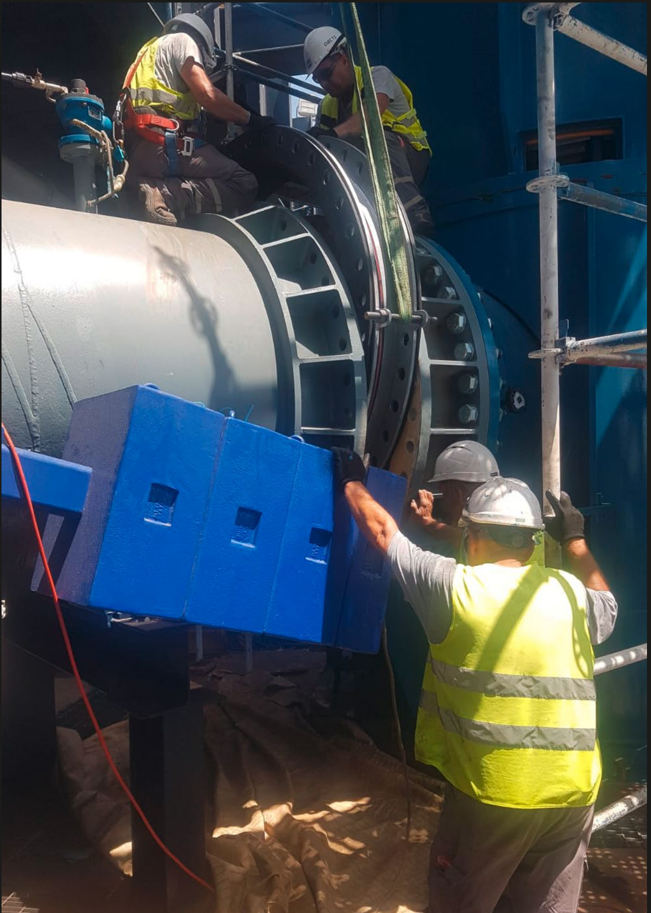
Installation of a rubber expansion joint \varnothing 1,600 mm to the pump nozzle, 16 bar design pressure
