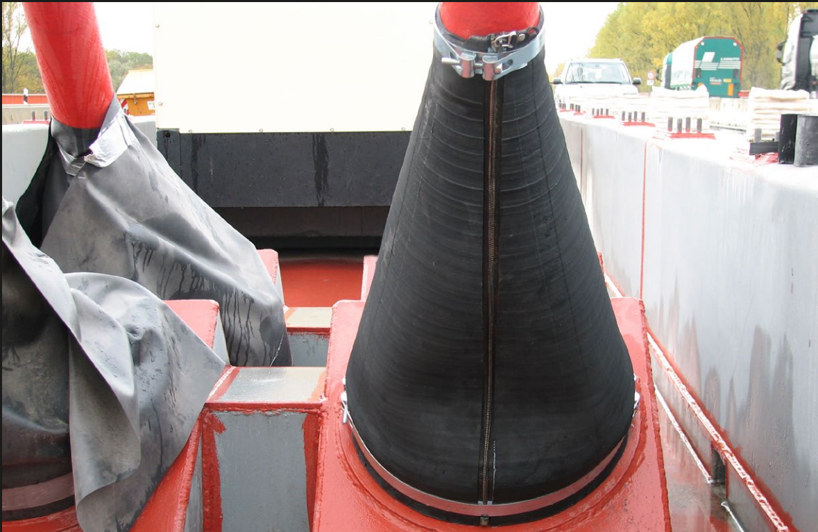
Concentric reducing expansion joint with zipper for maintenance service
