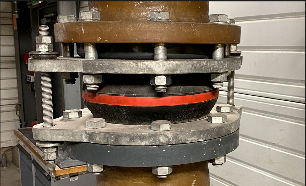
Single arch swivel flange EPDM rubber expansion joint to compensate lateral movements of a GRP pipeline
