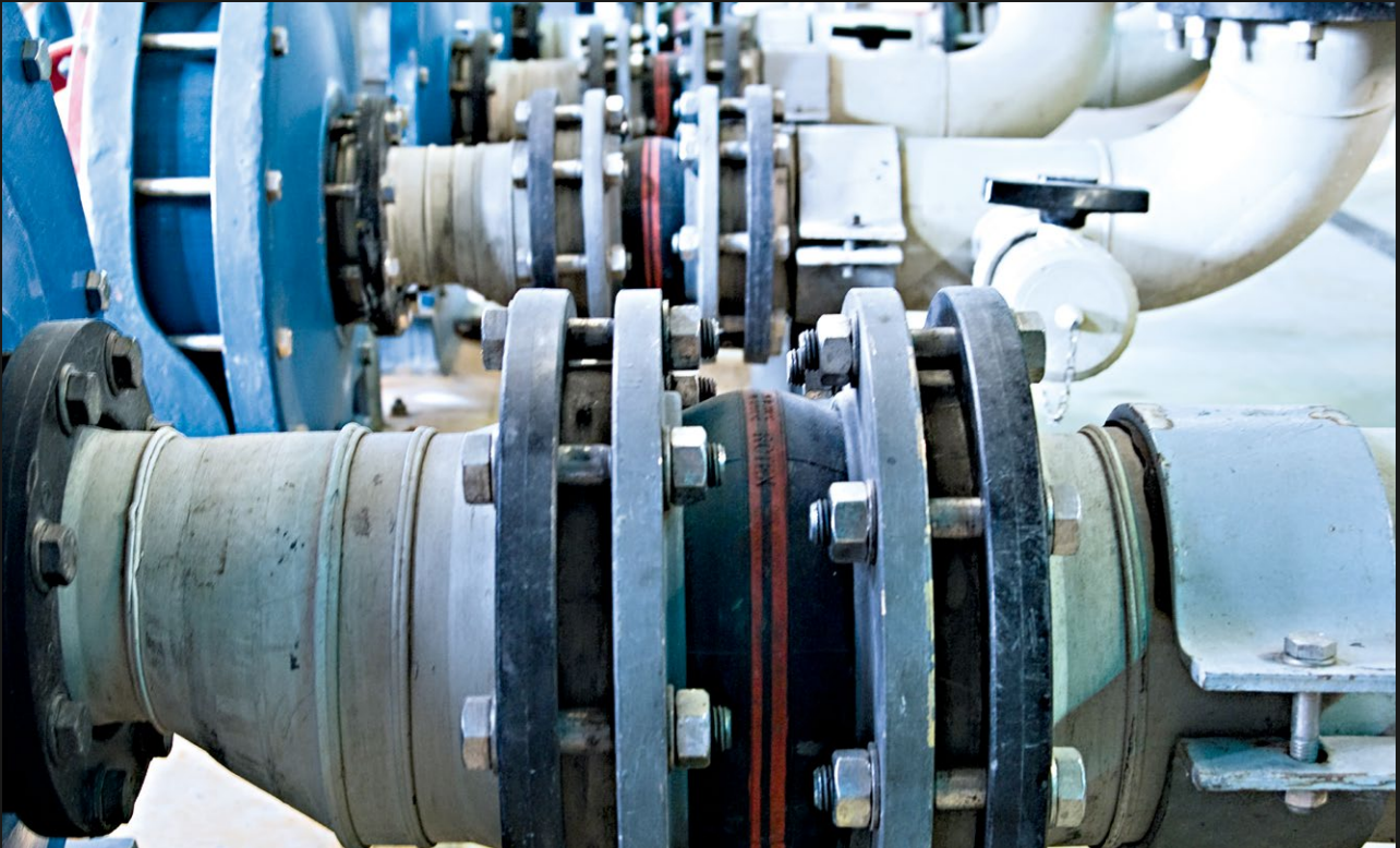
Universal expansion joint, type D110A on the suction side of quenching water pumps in a waste incineration plant Ø 150 mm, 16 bar
