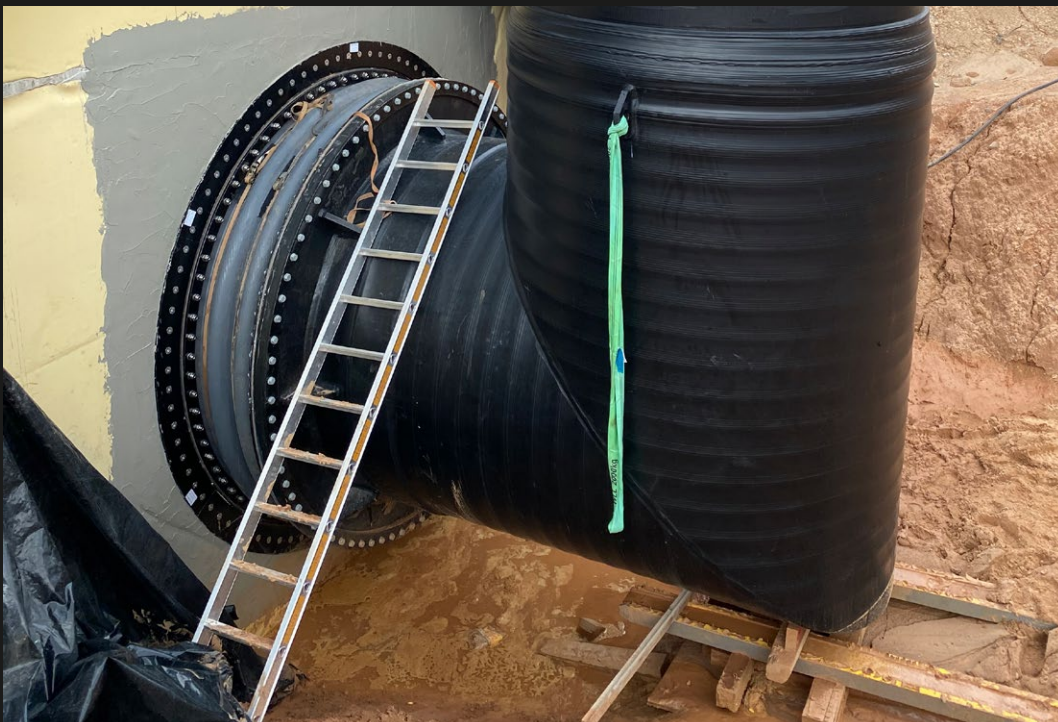
\varnothing 2,600 mm double arch ground water penetration seal made from radiation resistant silicone rubber installed outside of a building design pressure 20 m WC, lateral displacement 60 mm from building settlement
